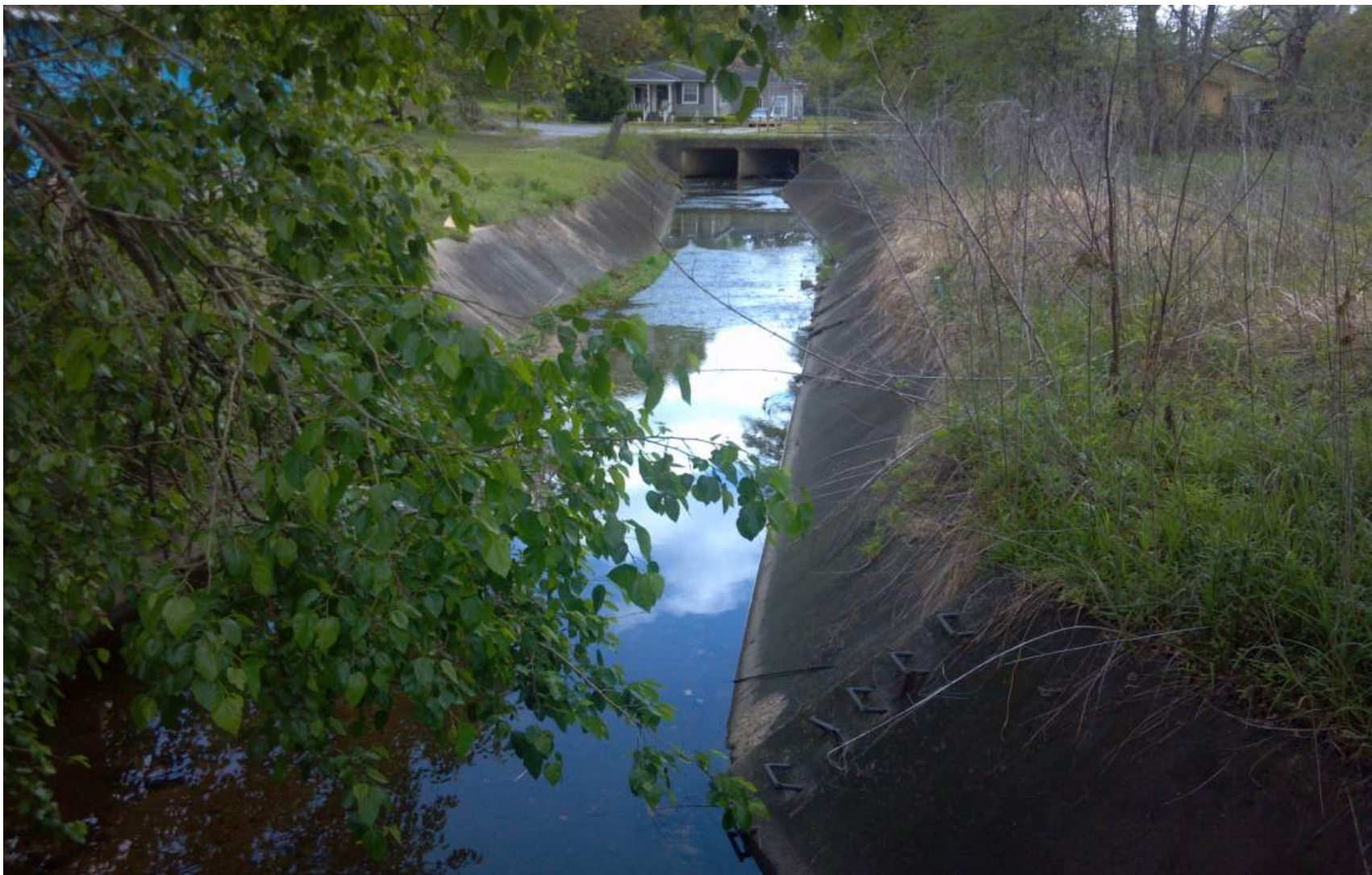
Figure 3-10 Concrete lined channel on Toulmins Spring Branch prohibits infiltration increasing stormwater runoff volumes and pollutant loads to Three Mile Creek, degrading water quality and habitat (Location: Toulmins Spring Branch downstream of Prichard Avenue)
