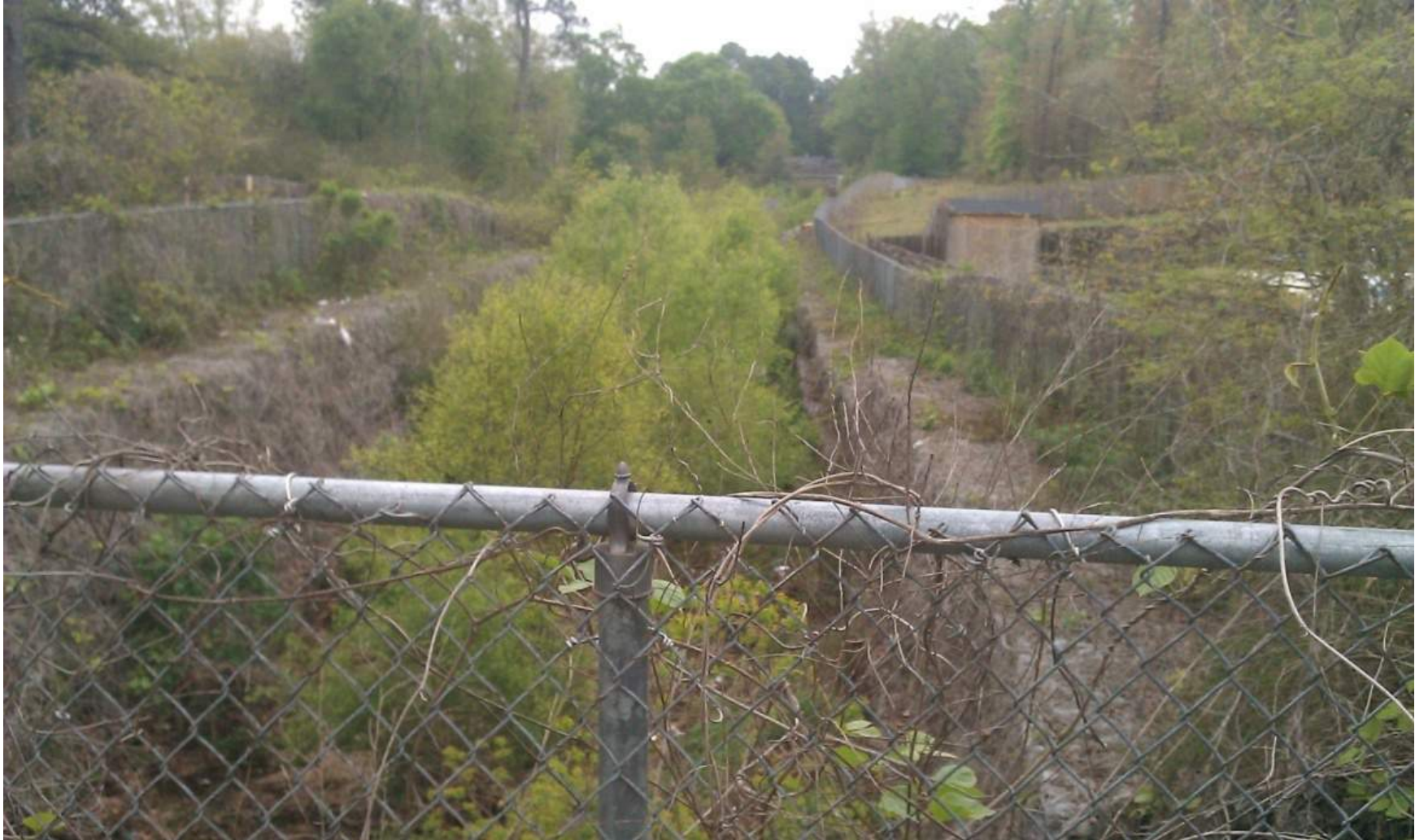
Figure 3-11 Gabion lined channel filled with sediment and vegetation reduces system drainage capacity and can result in localized flooding in the watershed (Location: TWEM downstream of Renn Street)
