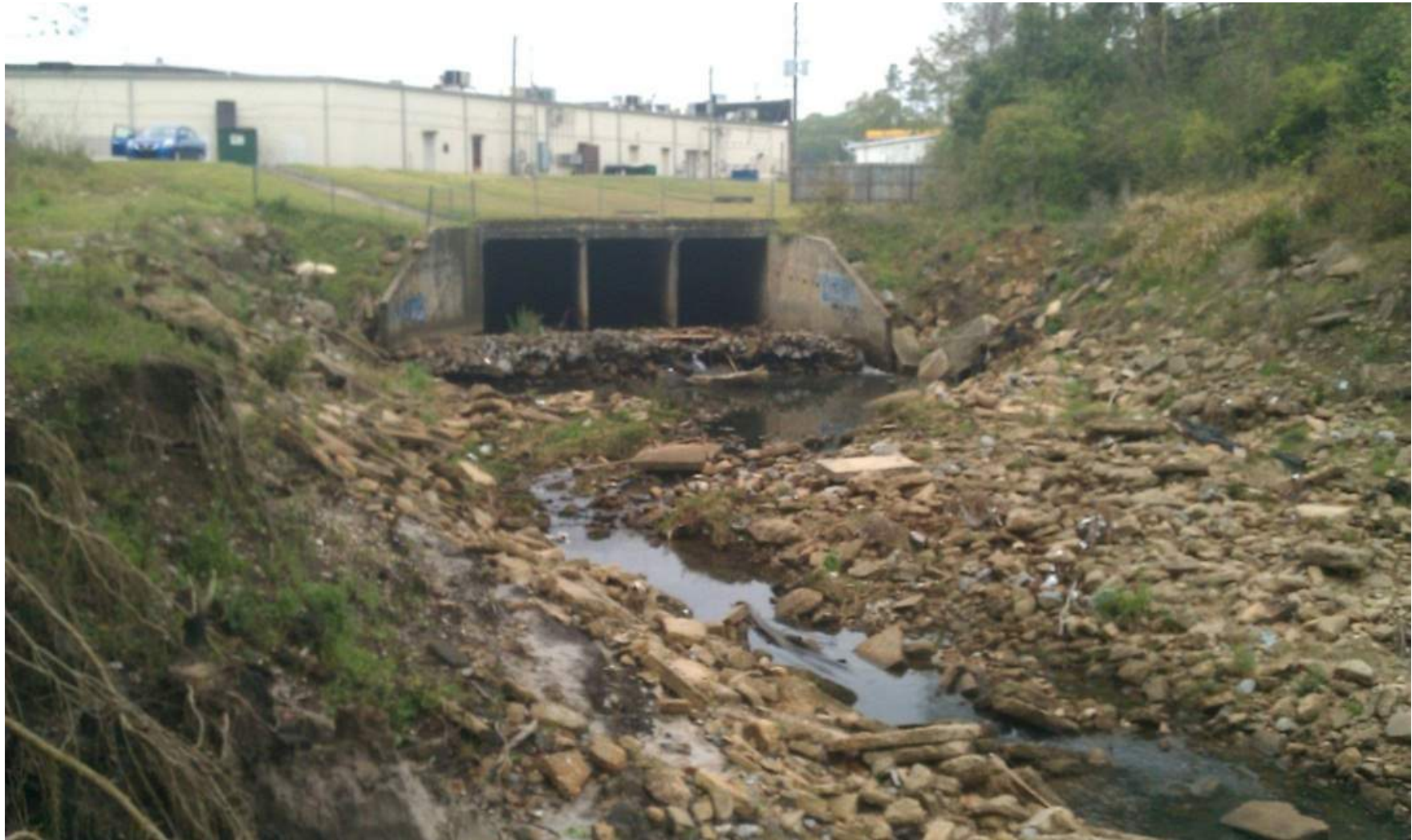
Figure 3-14 Erosion downstream of University Blvd in Twelve Mile Creek which flows into Three Mile Creek.
