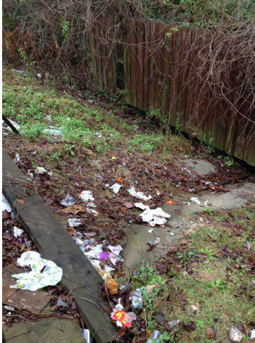
Figure 3-23 Gross Pollutants discharging from a dumpster pad via a concrete flume to a tributary to Three Mile Creek, degrading surface water quality and habitat (Location: Dollar General on Spring Hill Road)
