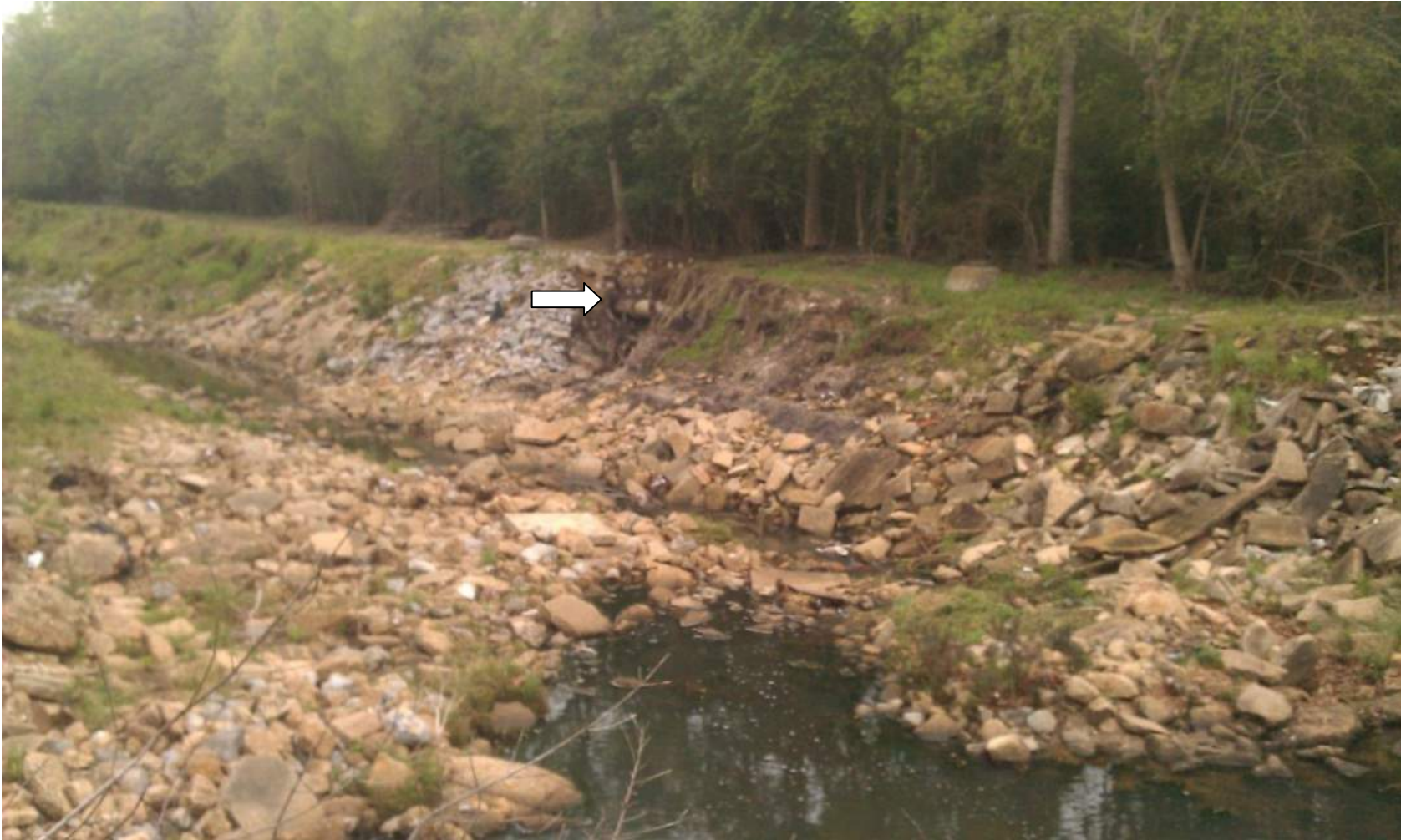
Figure 3-15 Exposed sanitary sewer pipe in Twelve Mile Creek from side stream erosion increasing the risk of a sanitary sewer leak into Three Mile Creek.
