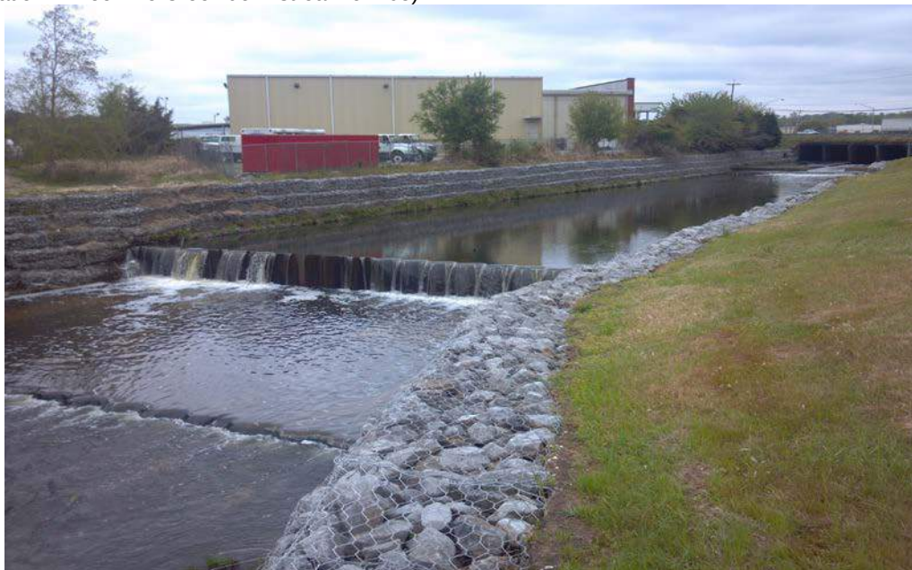
Figure 3-5 USACE channel widening and straightening, and installation of weir structures and gabion walls substantially changed the hydrology, hydraulics, water quality, and habitat of Three Mile Creek (Location: Three Mile Creek downstream of I-65)
