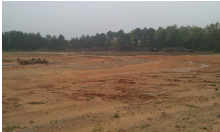
Figure 3-24 Undeveloped, exposed site near Cody Road and Zeigler Road with no construction site BMPs releases sediment and turbidity to Three Mile Creek, degrading surface water quality and habitat
