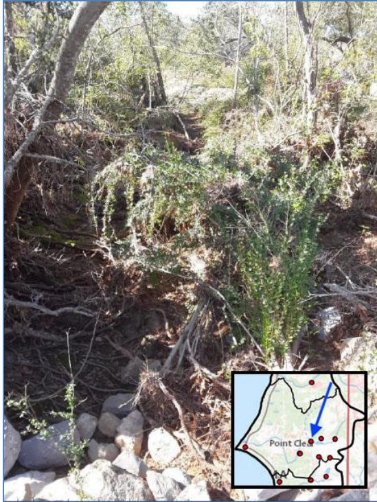
Figure 4.20 Eroded watercourse with a headcutting drain along Point Clear Creek at Section Street.
