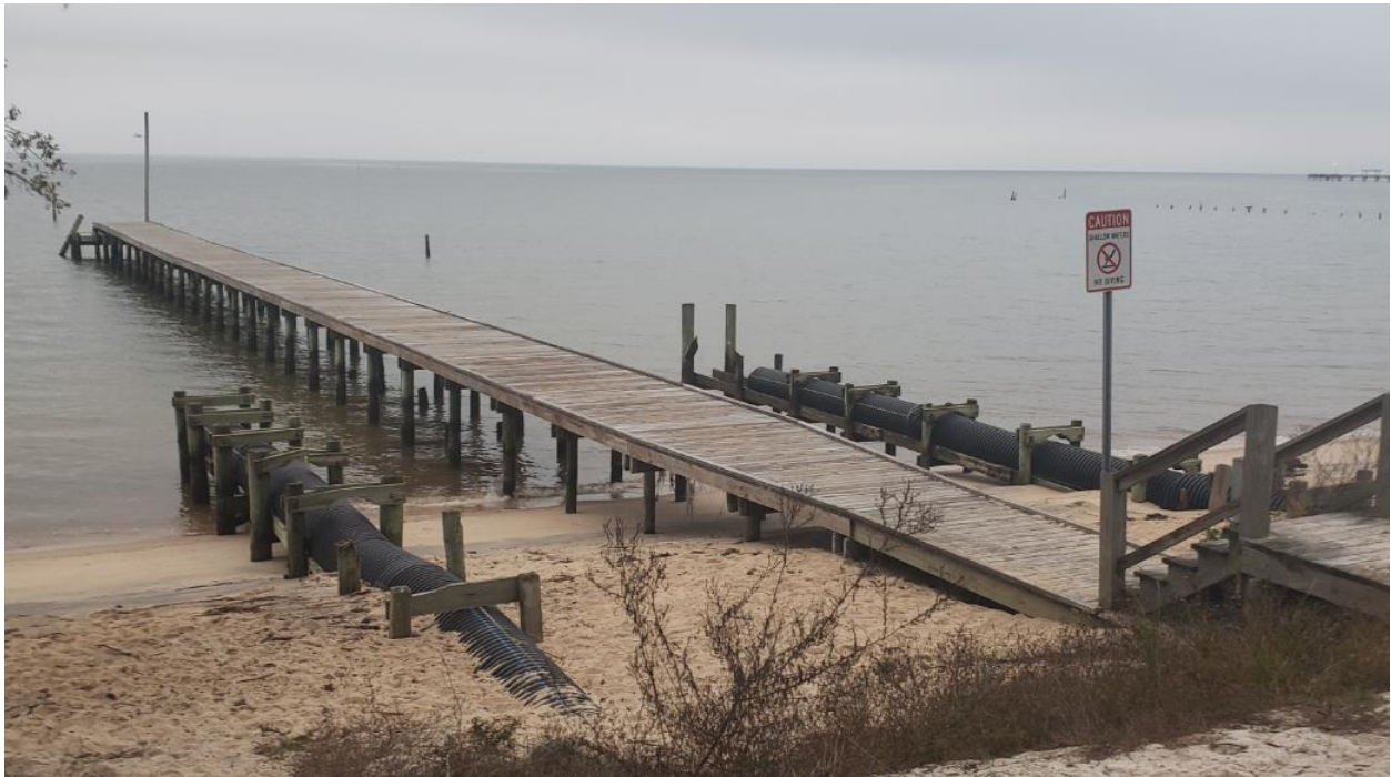
Figure 5.6 Example of Storm Drain that Could be Impacted by High Tail Waters
