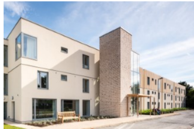
Rochestown House - Social Housing Project
