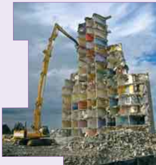
Demolition of Pearse Tower (2004)
