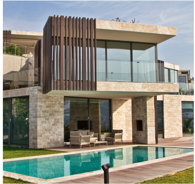
Technowood Profile Façade in Adres Yalikavak Villa
