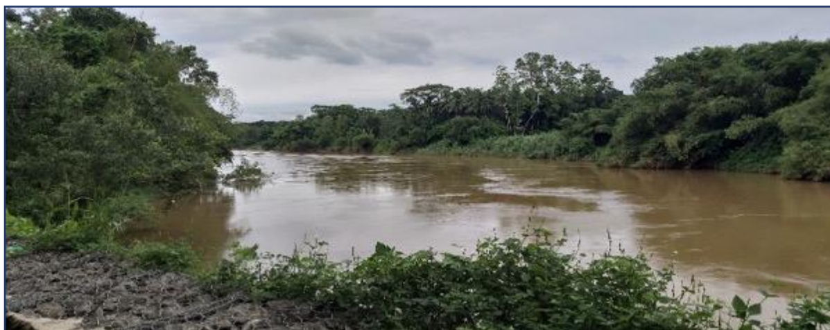
Figure 54: A gabion structure put along a section of river bank
