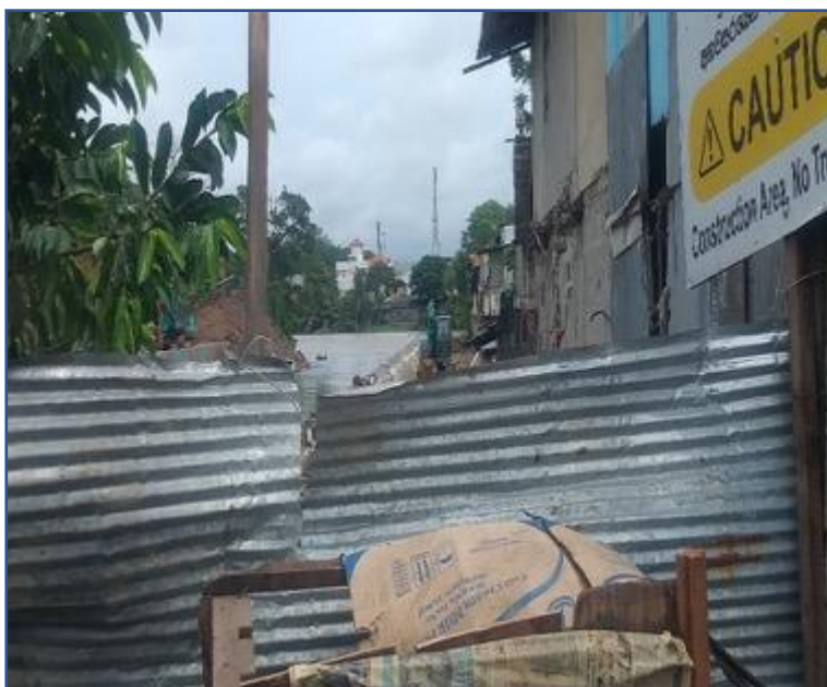
Figure 41: Rehabilitation works of St. Sebastian canal out fall at Kelani river
