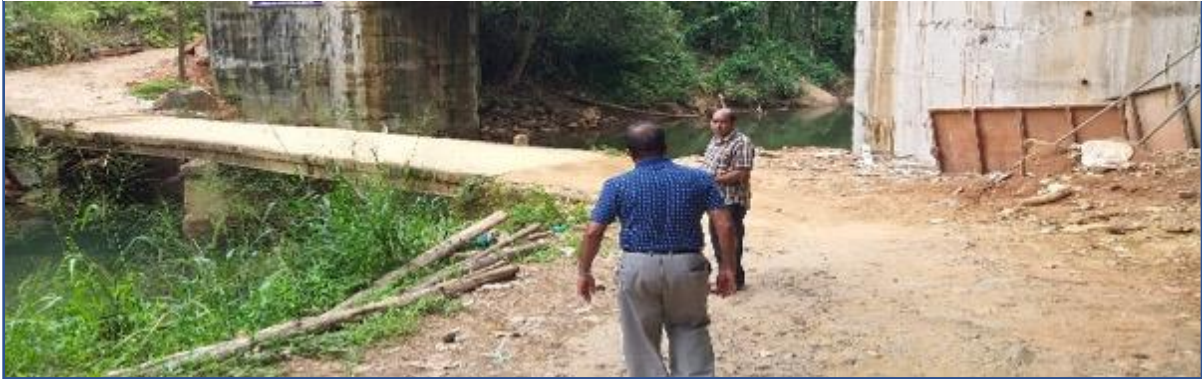
Figure 55: A new bridge being constructed across Magal Oya
