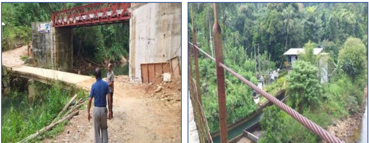
Figure 43: The new bridge under construction and the mini-hydroelectric power plant
