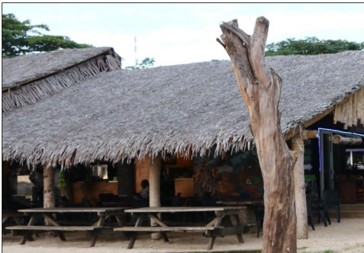
Figure 5.9 Roof thatching, Port Vila
