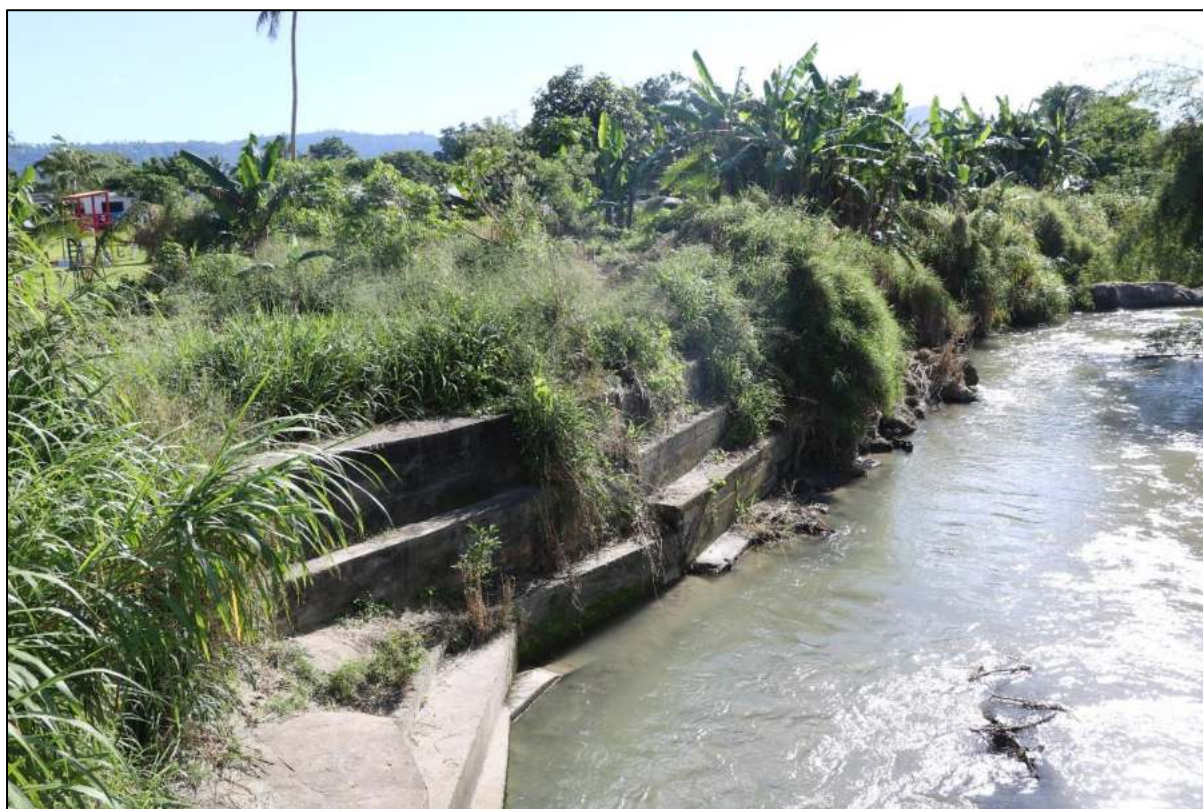
Figure 3.1 Typical river in urban reaches of Port Vila (near Mele)
